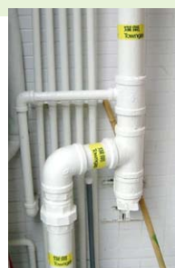
Figure 1: Vertical sections of a service riser
