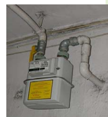
Figure 3: An installation pipe and gas fittings
