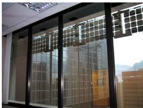
Figure 4: Sunshade Sub-system – Interior View
