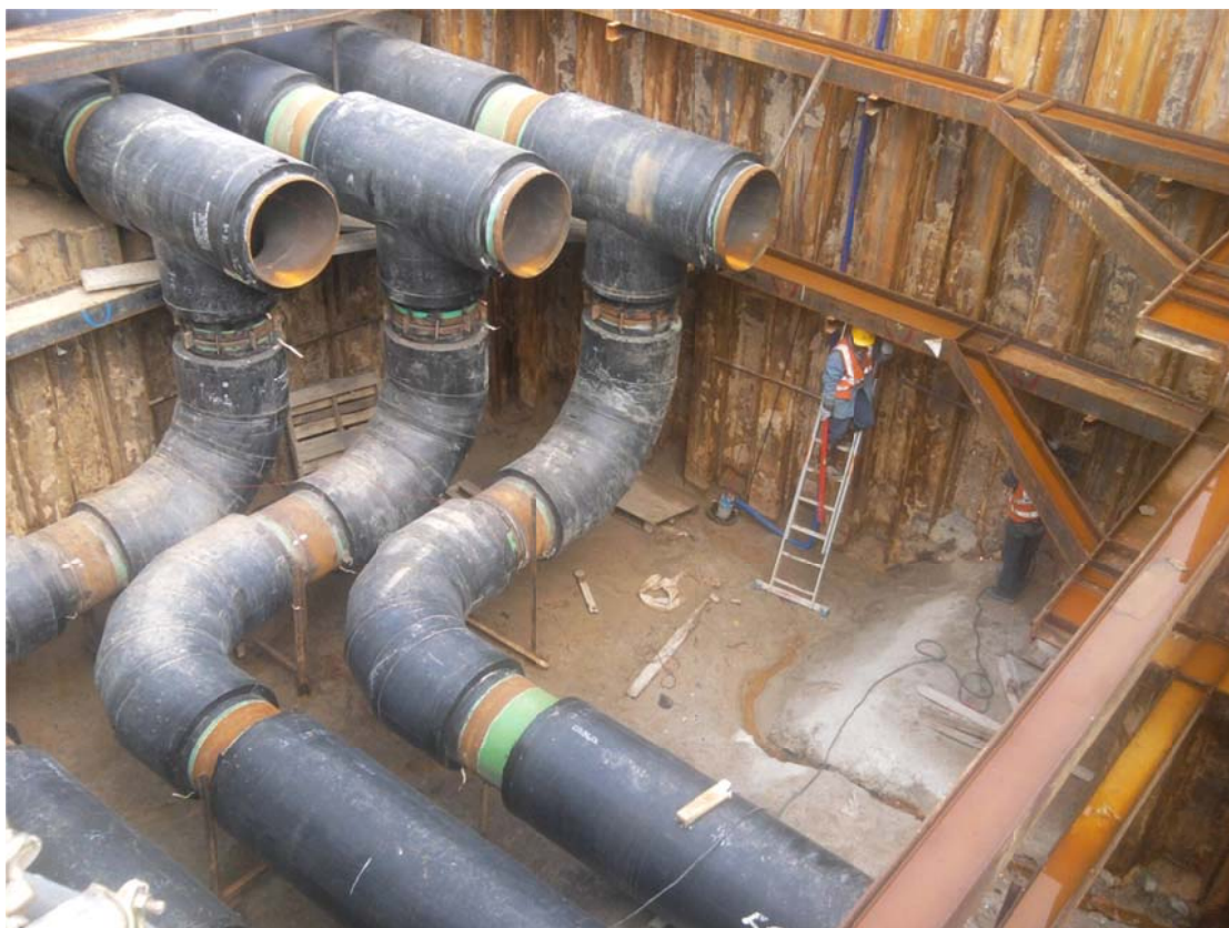
Figure 3 - Grout curtain and dewatering provided at deep open trench for pipe laying
