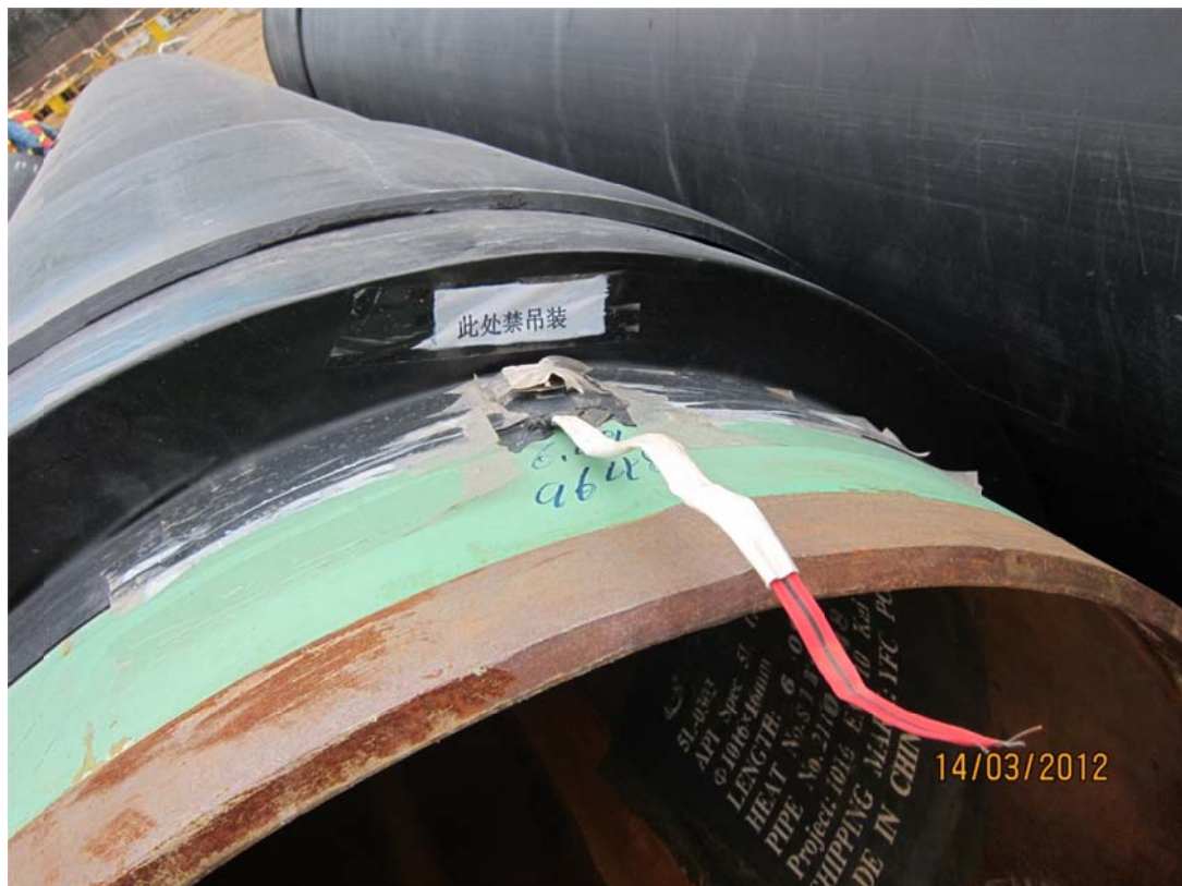
Figure 2 - Prefabricated chilled water pipe with leakage detection cables and polyurethane insulation with HDPE outer jacket
