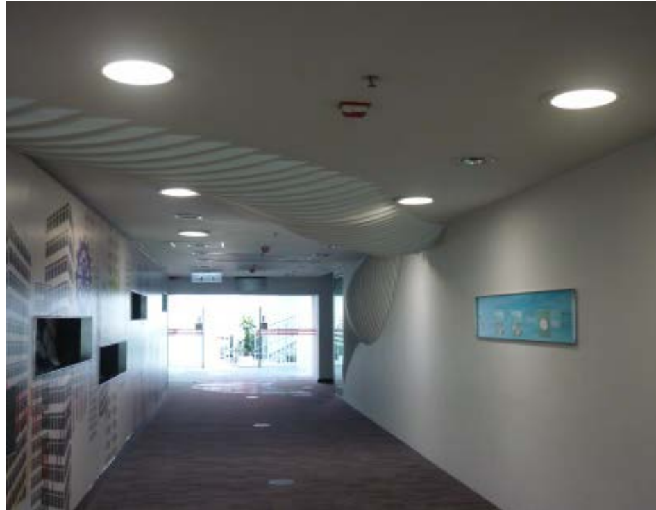
Corridor properly lit up by Sunpipes
