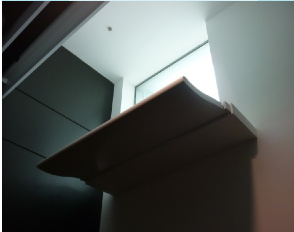
Corridor properly lit up by Sunpipes
