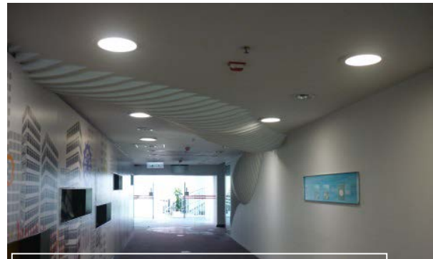
Figure 5 : Corridor properly lit up by Sunpipes
