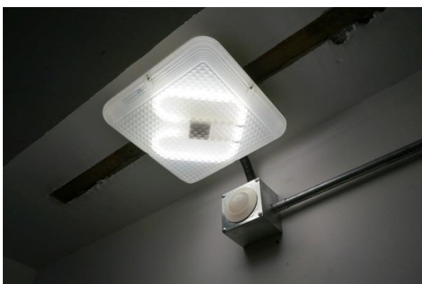
Fig. 10 Motion Sensor for Lighting Control
