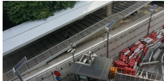
Fig. 7 LED Solar Compound Lighting
