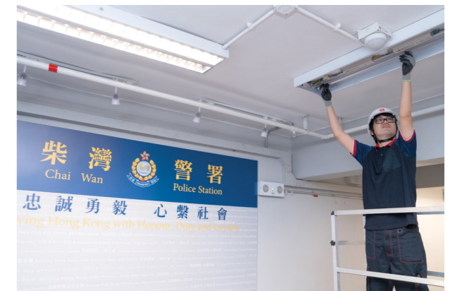
我們把柴灣警署現有的照明燈具更換為節能的發光二極管燈。We replaced the lighting at the Chai Wan Police Station with energy-efficient LED lights.
