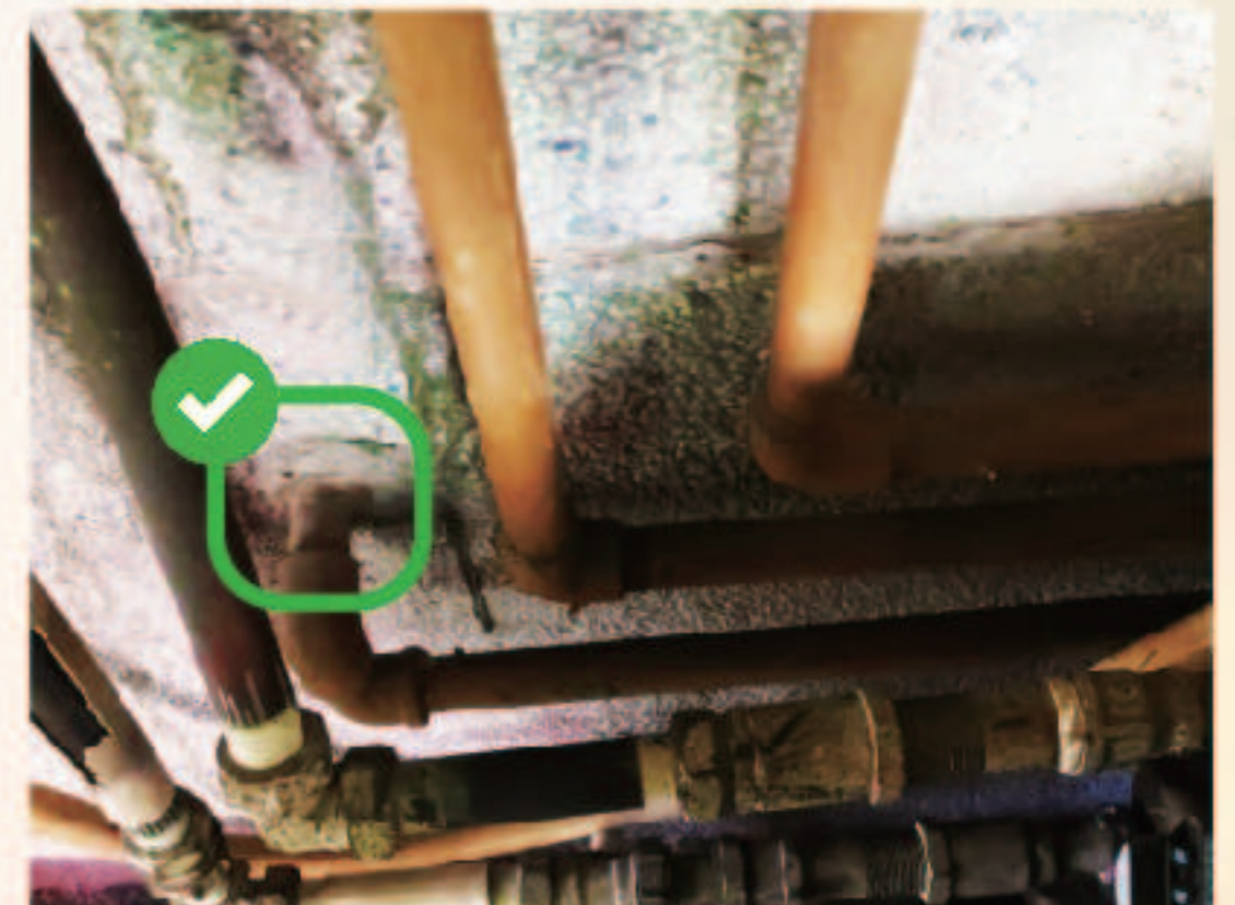
✓ Using a metallic gas pipe to pass through an external wall
