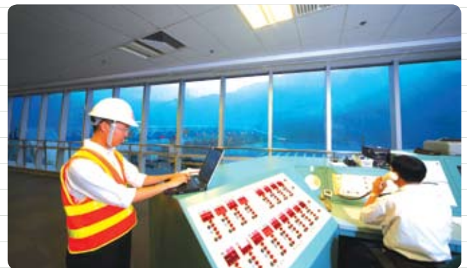
測試八號幹線控制中心的交通控制系統，確保交通流動暢順。 Testing the traffic control system at Route 8 Control Centre to ensure the smooth flow of traffic.
